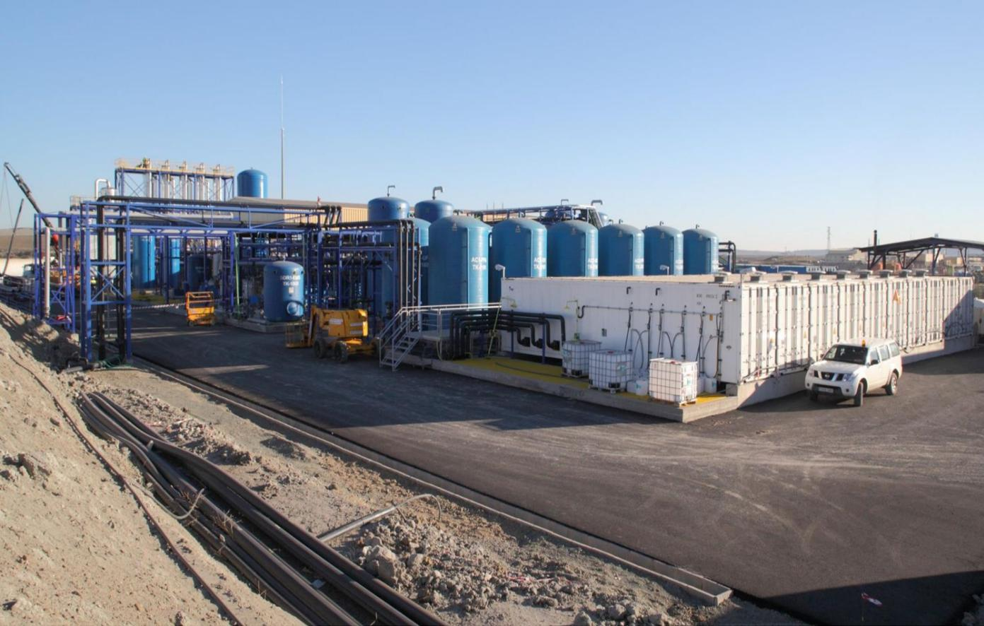
Treatment plant for Contact water from a Copper mine, Membrane area 10.000m<sup>2</sup>, 95% recovery
